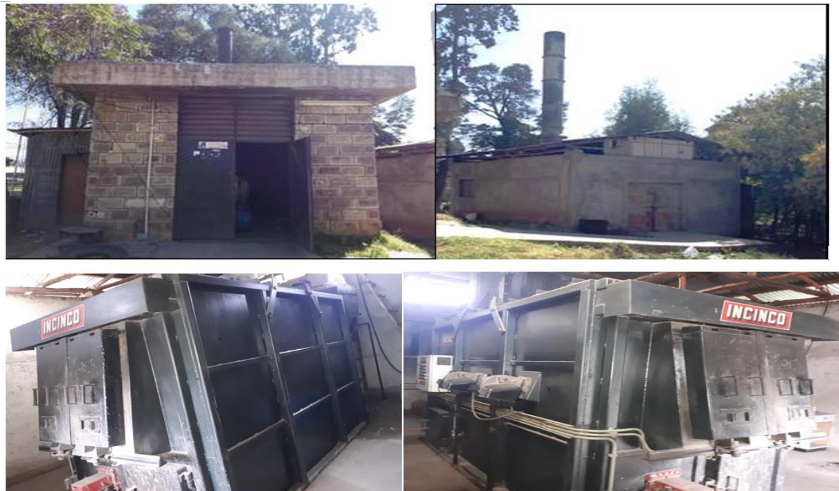
Figure 9: Incinerators at EPHI for Waste Management
