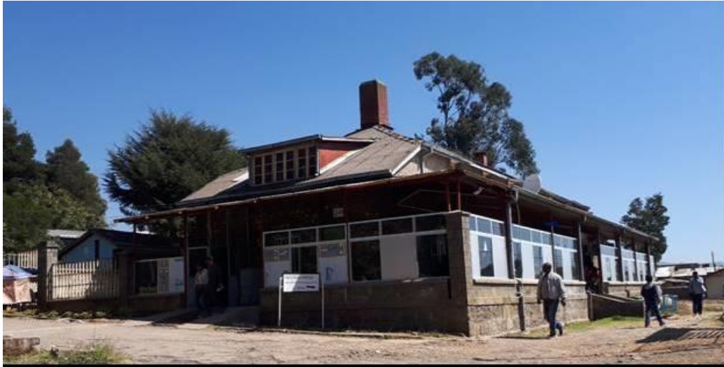
Figure 16: Sample collection Building near the laboratory
