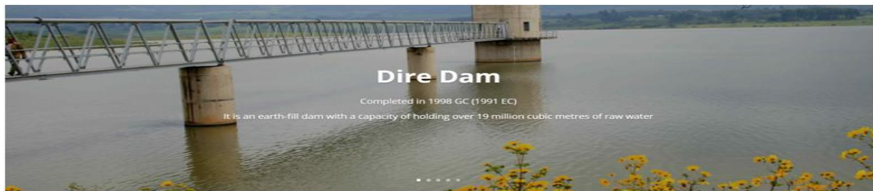
Figure 13: Dire Dam and Treatment Plant
